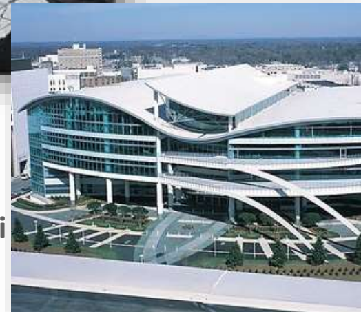
Roofing membrane (TPO)
